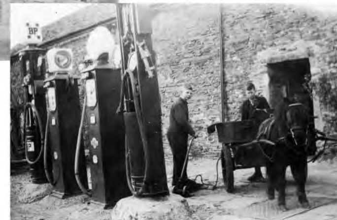
Soon after, the BP pumps were installed. Gordon and Joseph Norman, casual employees, inflate a tyre.
