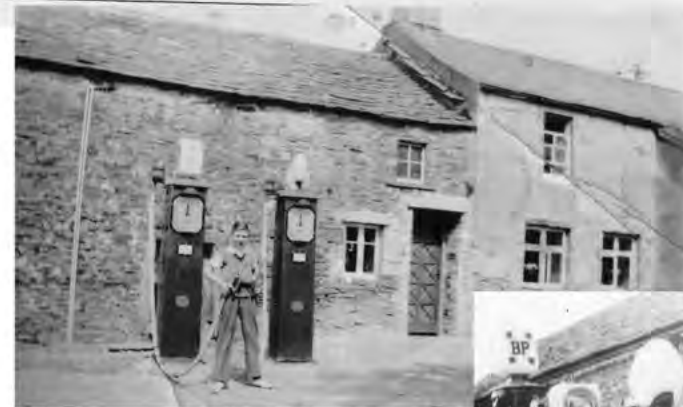
Gordon Norman, an occasional helper, with the newly installed first two pumps in 1937/8. While there are two brands, National Benzole and Shell, these two companies had merged in 1932.
