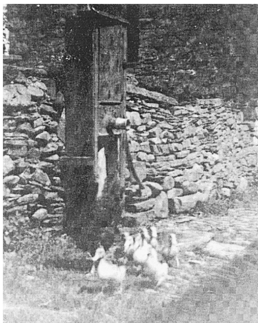
The old pump, 1950s
