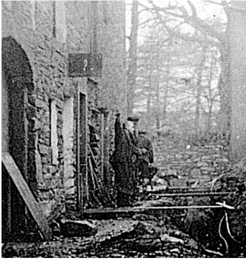
The ? shop sign in 1938, laying sewers
