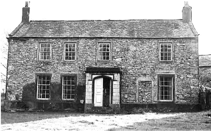
Rendering removed from the front façade, showing the blocked-up doorway, 1978
