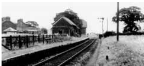
Embleton Station; image courtesy of Eric Cass.
